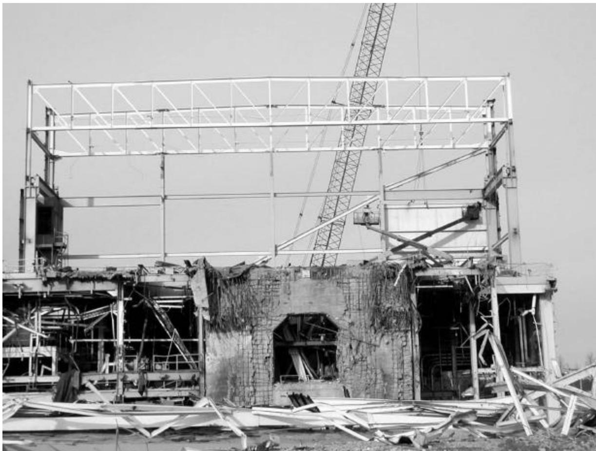
**Figure 7-7 Turbine Building Demolition After Use of Explosives**
