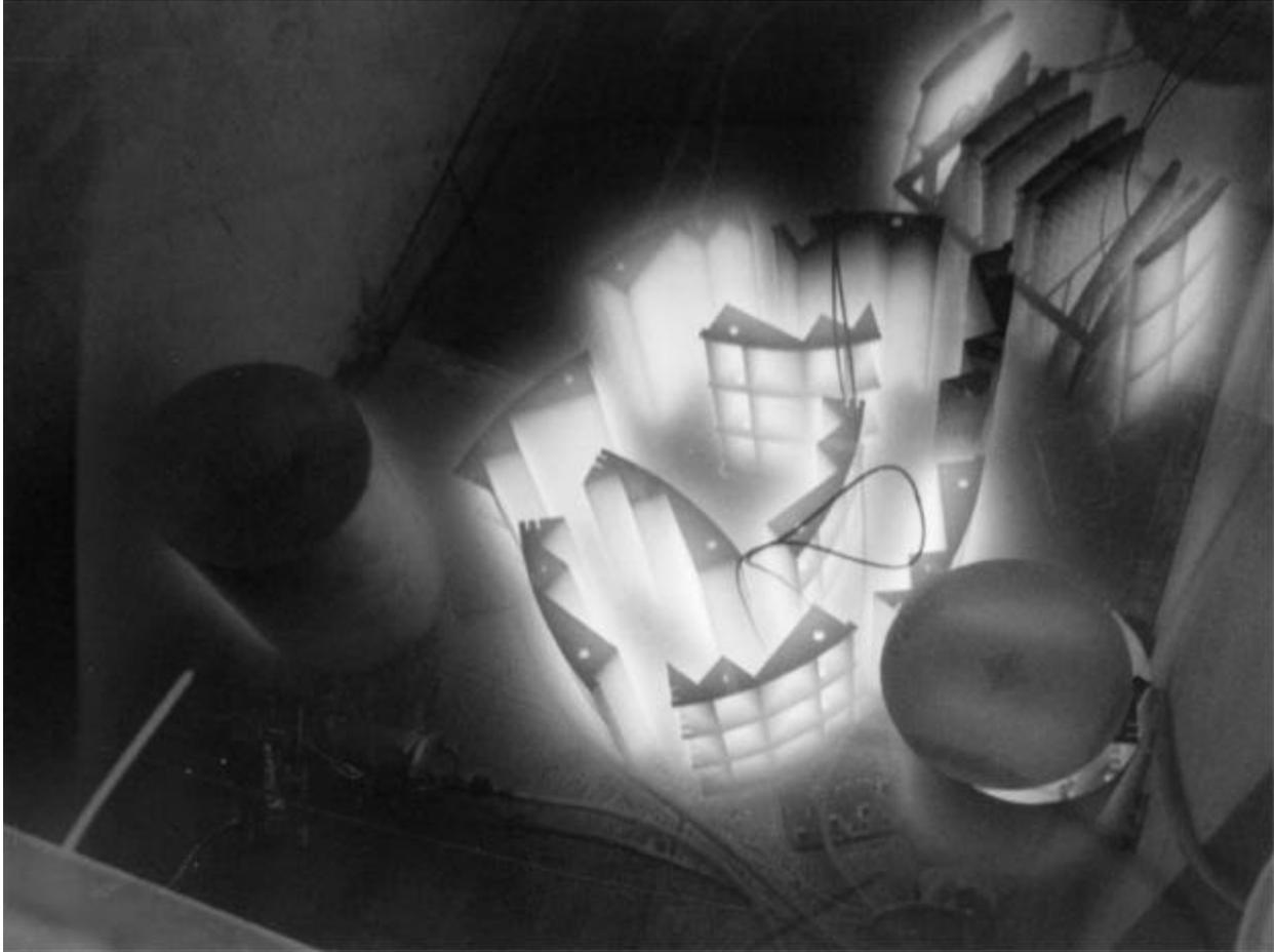
**Figure 7-3 Maine Yankee Vessel Internals Segmentation**
