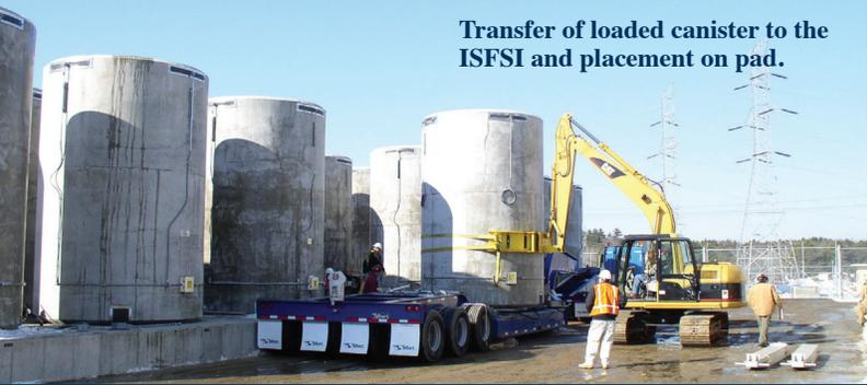
Transfer of loaded canister to the ISFSI and placement on pad.
